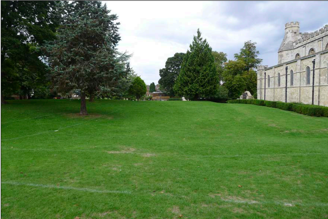
Figure 15: The sub-square hollow [2] indicating the former location of the cloister to the south of the church, view looking west. 12-SEP-2022. © Historic England
