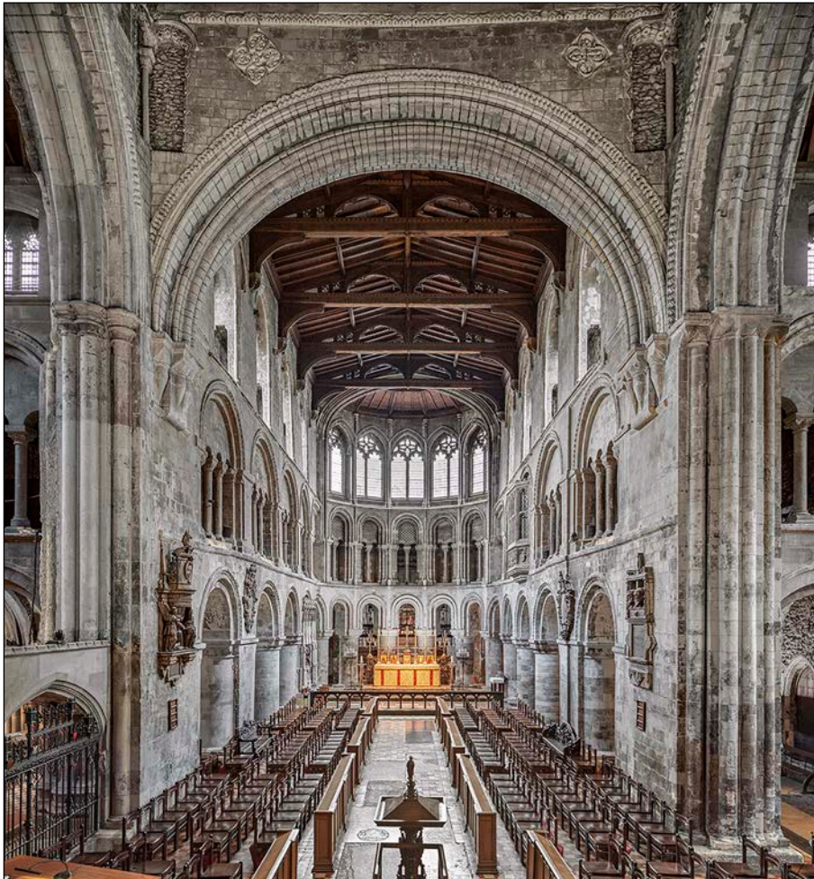
Figure 29: The eastern end of St Bartholomew the Great, Farringdon, London, with rounded apsidal end and arcaded ambulatory. Image: Chris Redgrave DP462404 © Historic England Archive.
