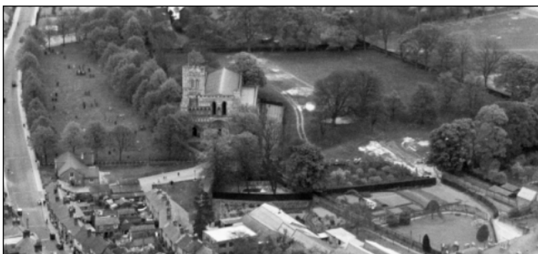
Figure 19: Extract from a 1938 aerial photograph showing the insertion of a service pipe across Priory Gardens, looking east. EPW056929 26-APR-1938 (Historic England Archive: Aerofilms Collection)
