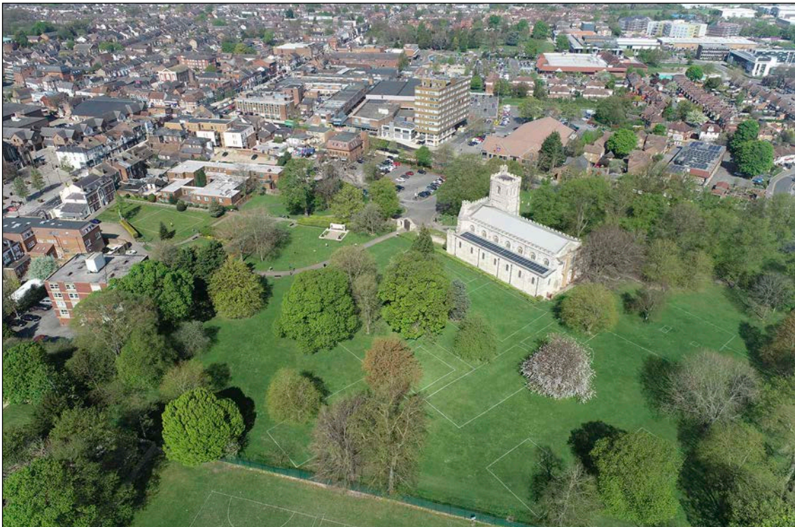
Figure 1: Priory Gardens (looking north) with the Priory Church of St Peter (centre right) and Priory House (centre left). The white lines painted on the grass are an interpretation of the probable positions of the priory buildings based on geophysical surveys. Photograph: Matthew Bristow 21-APR-2022
