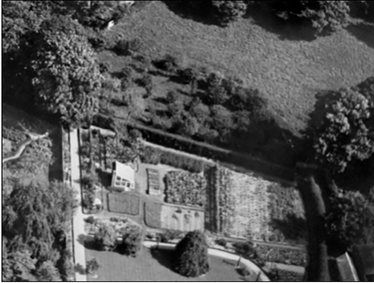
Figure 25: Detail from a 1928 aerial photograph of the kitchen garden area and orchard beyond, looking north-east. EPW023862 01-SEP-1928 (Historic England Archive: Aerofilms Collection)
