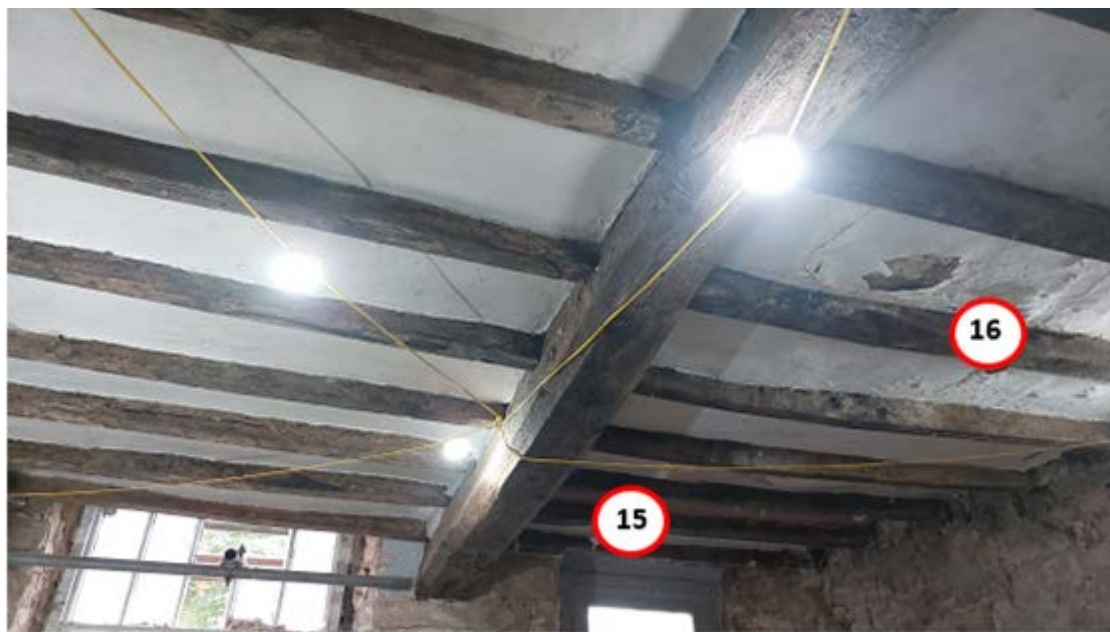
Figure 3h: North Cottage, north bay, viewed looking northwest. [photograph Robert Howard]
