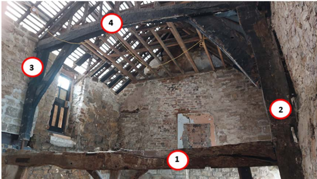
Figure 3a: South Cottage, truss 1, viewed looking south. [photograph Robert Howard]
