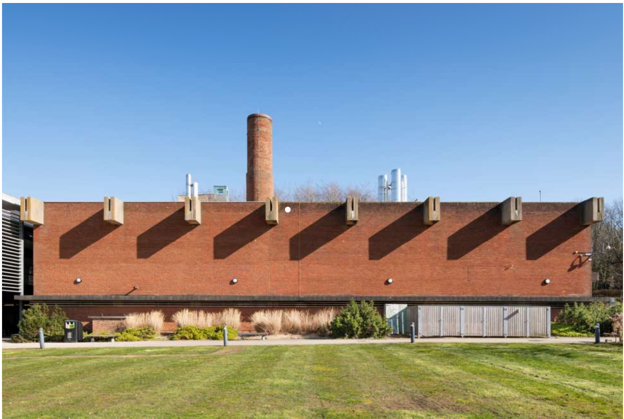
Boiler House designed by Sir Basil Spence, University of Sussex, Brighton, East Sussex. Included on Brighton and Hove’s Local Heritage List. James O. Davies © Historic England Archive DP439659
