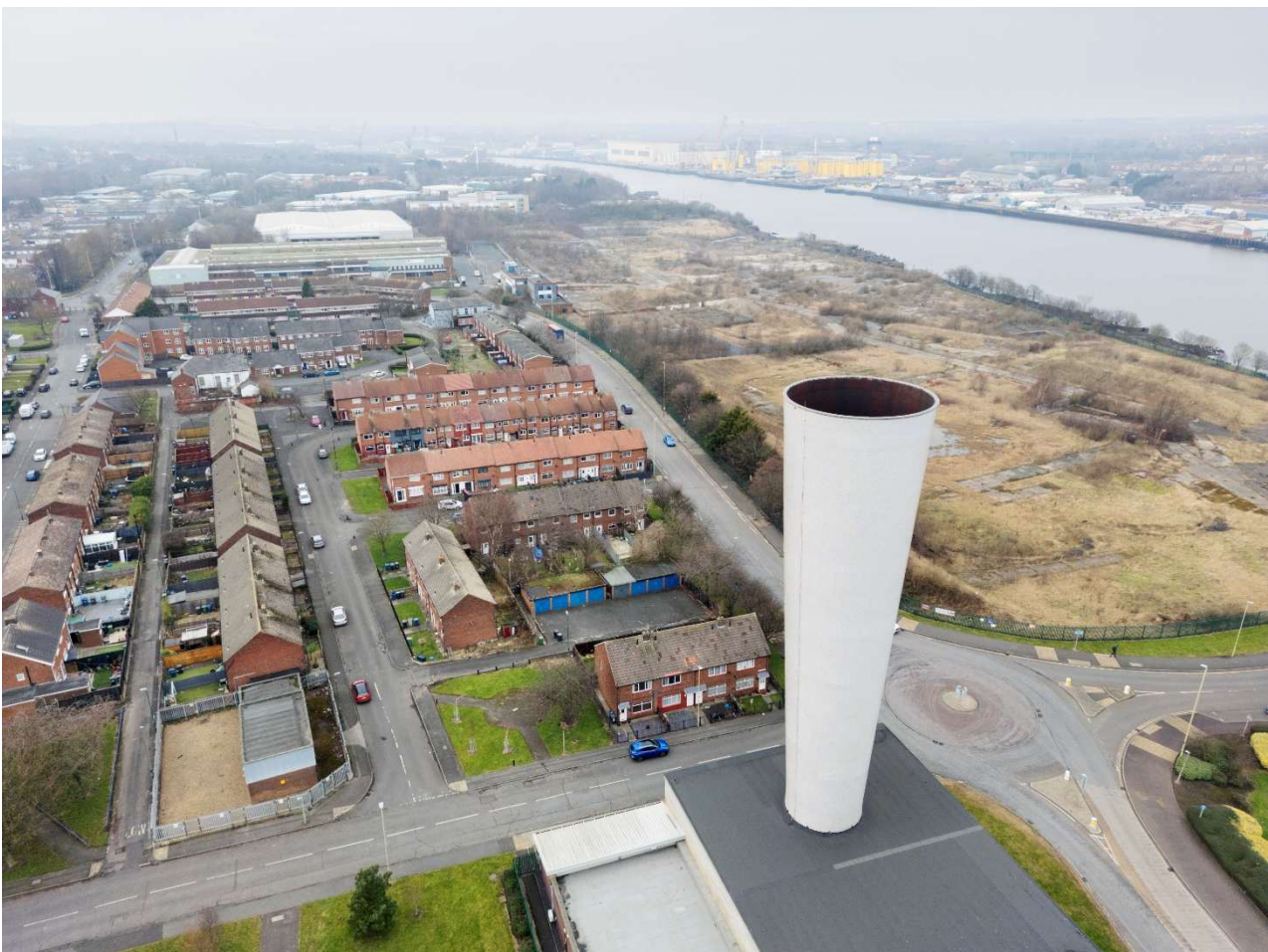
Tyne Tunnel Ventilation Tower (South Side), Ferry St/Chaytor St, Jarrow, Tyne & Wear. Included on South Tyneside’s Local Heritage List. Alan Bull © Historic England Archive DP486725
