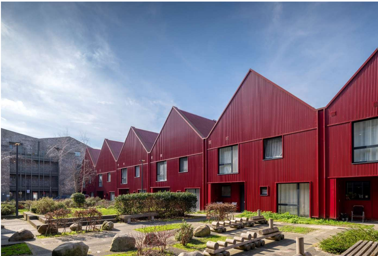
Sutherland Road affordable housing scheme by Levitt Bernstein, Sutherland Road, Waltham Forest, London. Included on the London Borough of Waltham Forest's Local List. Chris Redgrave © Historic England Archive DP528483.TIF
