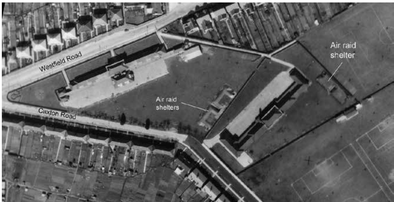
Figure 126: Two large air raid shelters at Garlinge Primary School still extant in 1951. [Extract of RAF/58/618 V 5089 11-APR-1951. Historic England Archive (RAF Photography)]
