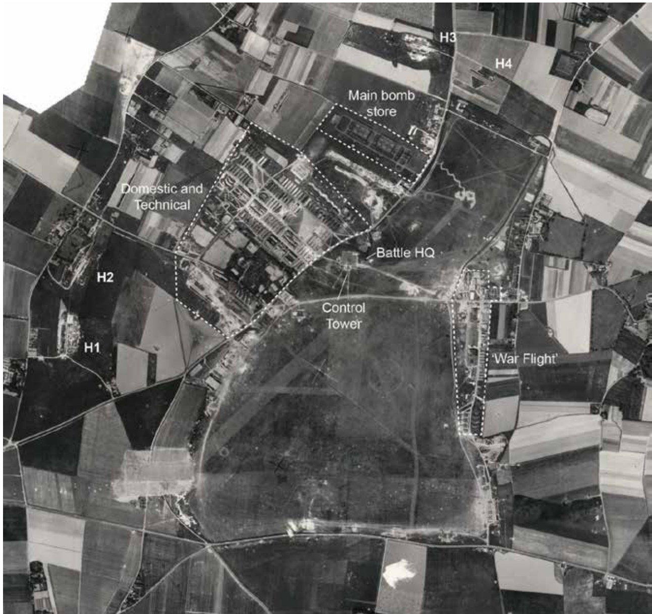
Figure 92: RAF Manston and immediate environs on 1 June 1942. Key areas brigaded around the airfield are outlined. Semi-sunken hangars: H1, Alland Grange; H2, Cheeseman's Farm; H3, Manston Road; H4, Manston Road (unfinished). North to top, unscaled composite image. [RAF/HLA/564 V 6012-16, 6020-1, 6027-9, 6033-8, 6041-5 01-JUN-1942. Historic England Archive (RAF Photography)]
