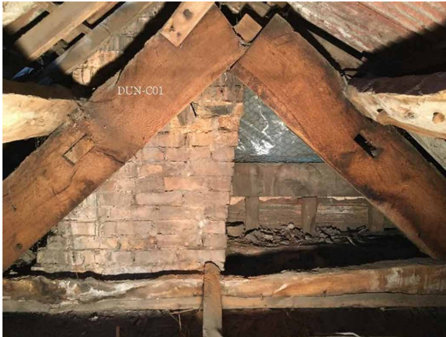
Figure 3: T1 is a true cruck. Sampled timber marked DUN-C01, photograph taken from the south. [Alison Arnold]
