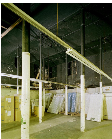
Figure 8. The internal boiler house.
