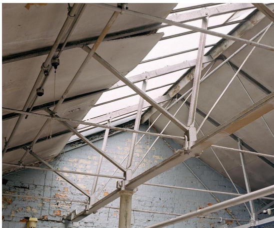
Figure 7. Angled struts, strut housings and inserted longitudinal beams.
