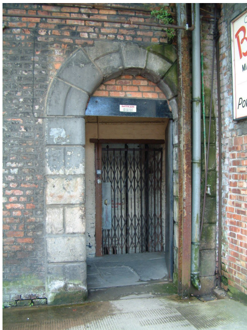
Figure 2. The main entrance to the stair and hoist tower.
