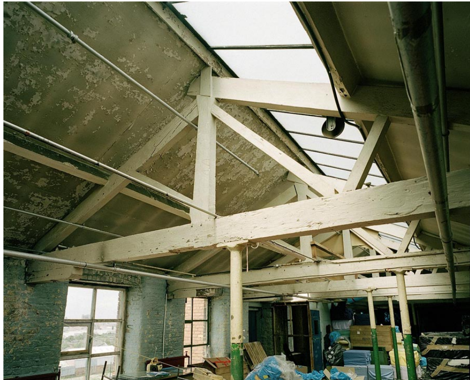
Figure 4. The west side of the timber roof.
