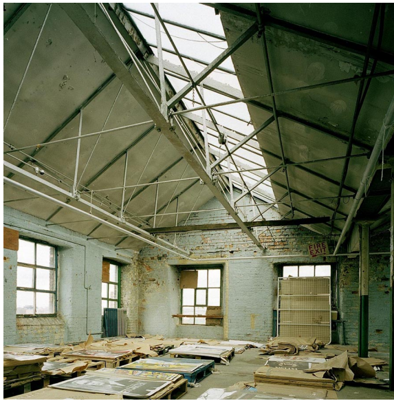
Figure 5. The west side of the iron roof.
