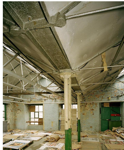
Figure 6. Detail of valley gutter, columns and Y-brackets.
