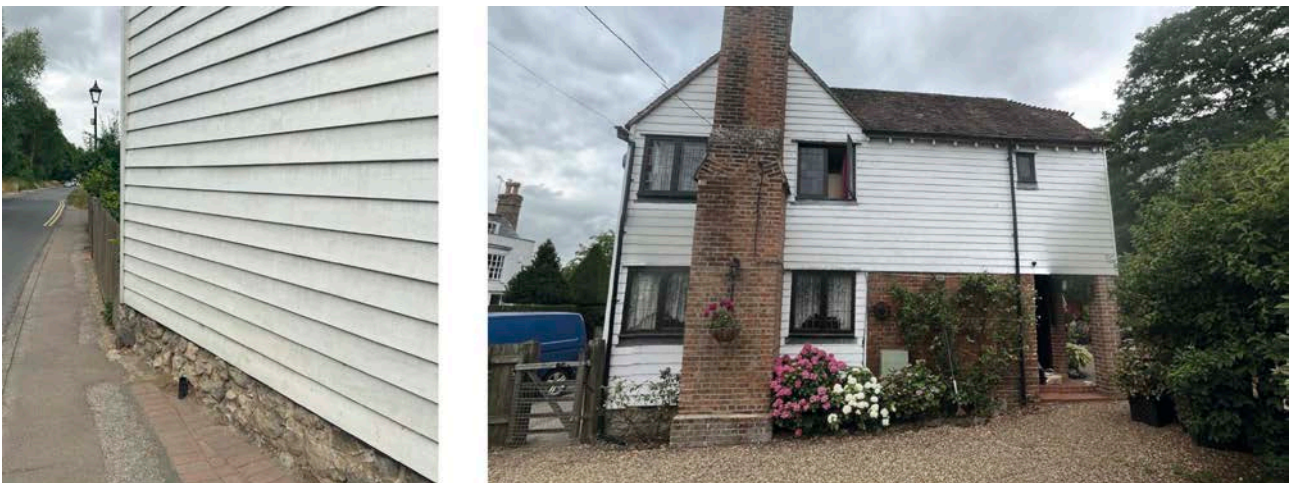
Figure 17: Cladding on Lees Cottage © The Environmental Design Studio
