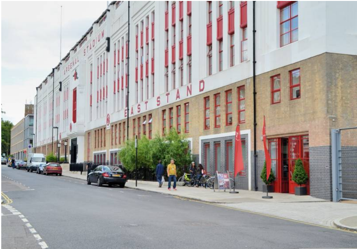
Figure 18 – Retained structure of former stadium at Highbury Park Now adapted as part of residential overhaul of Arsenal's former stadium © Licenced for reuse under CC BY-NC-ND 2.0
