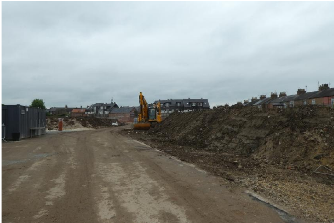
Figure 23 – Constructing 'David Longhurst Way'
