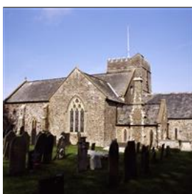
© John Warlow. Source Historic England Archive
